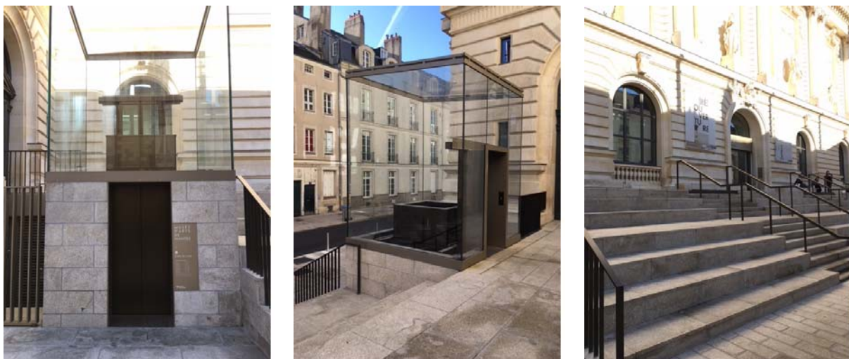
Figure 6, 7 and 8: External access points to the museum with a lift and handrails (Source: Author)
