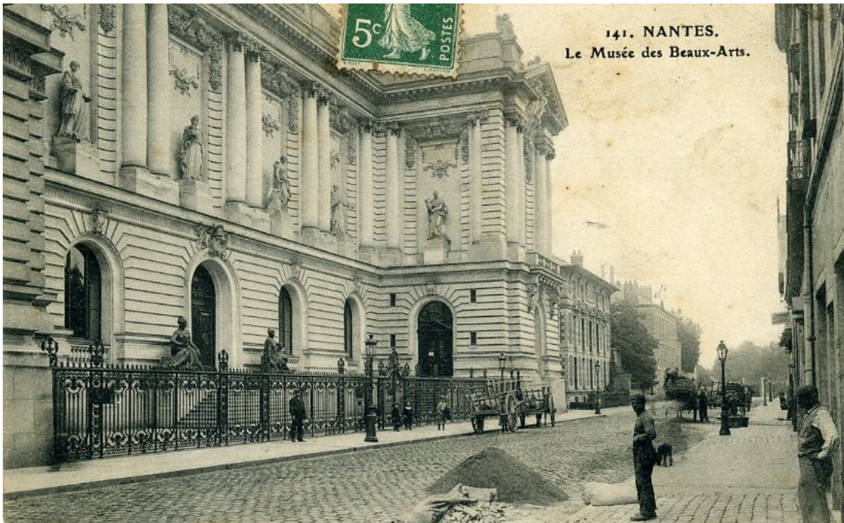
Figure 3: Palais des Beaux-Arts de Nantes, inaugurated in 1900 (Source: © Domaine Public)
